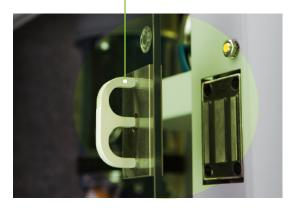
With a Pevco security door in place, hospital staff must enter an authorization code to release the durable electromagnetic lock to access the station's contents. Once unlocked, the door stays open, leaving hands free to remove the carrier that has arrived. If the door is not manually closed within 60 seconds, a programmable alarm rings as a reminder to close the door.
